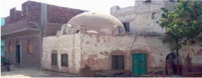
(Fig. 4) Remodeling New Gurna houses http://whc.unesco.org/en/activities/637/
